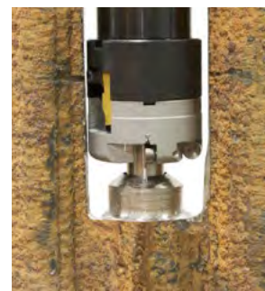
Remove membrane and overlay/cladding from between tubes
